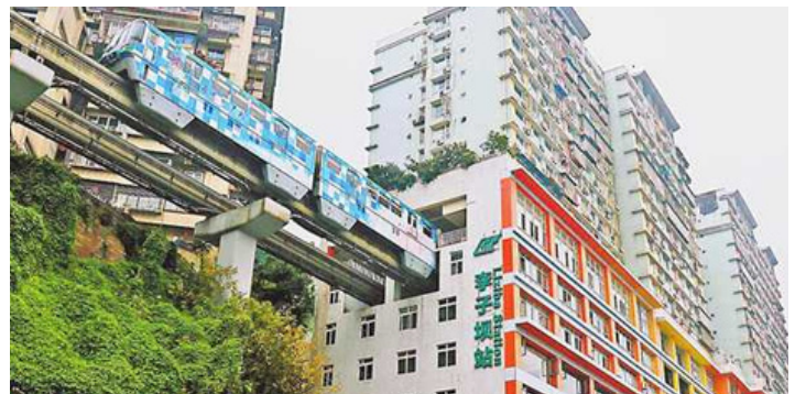
Liziba Light rail through the building
