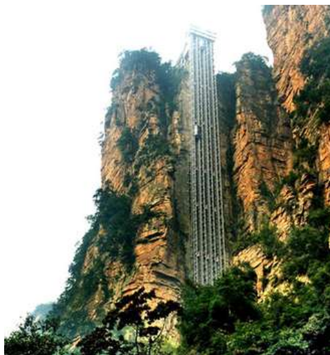
Zhangjiajie BAILONG ELEVATOR 百龙天梯
